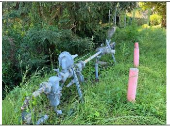
Photo: Gas Meter on North Side of River
