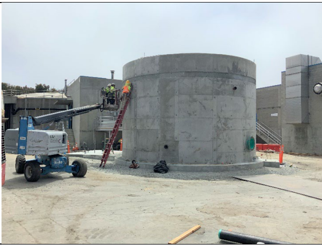
Photo: New Sludge Tank Under Construction
