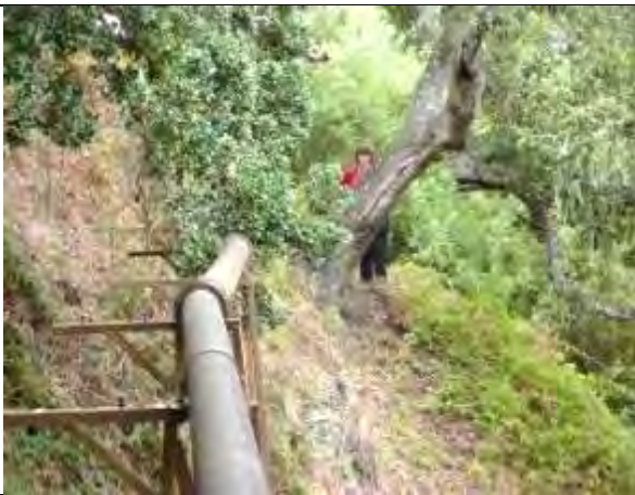
Photo: View gravity pipe in Carmel easement
