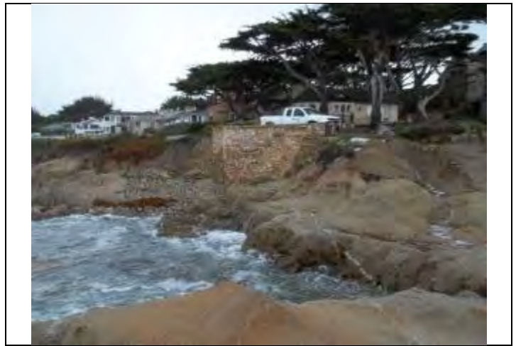
Photo: Looking at Pump Station Exterior
