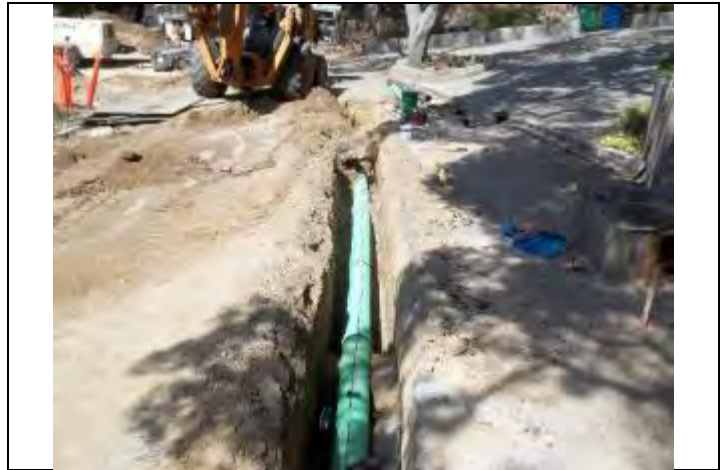
Photo: Sewer Line Repair
