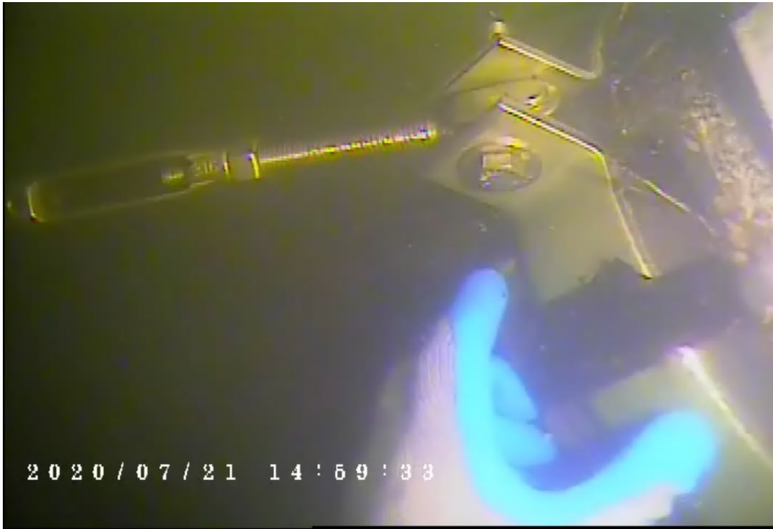
Image 5 – Upper clamp-to-turnbuckle connection of soft reaction bracing (typical)
