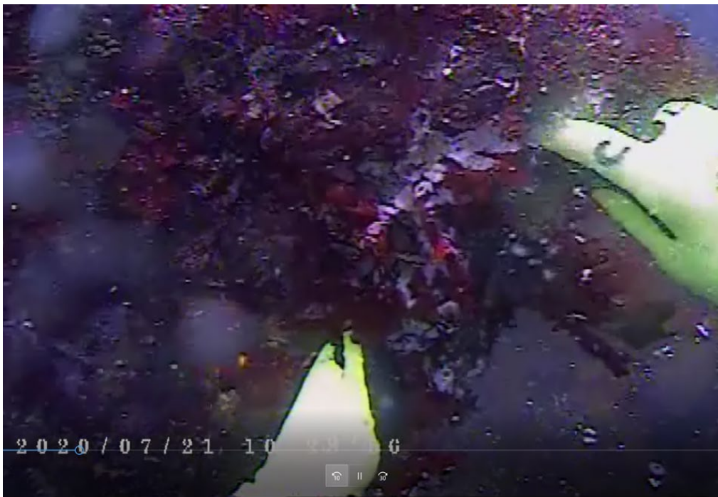
Image 1 – Duckbill contact sealing surface during no-flow (Screen capture taken from diver video track)
