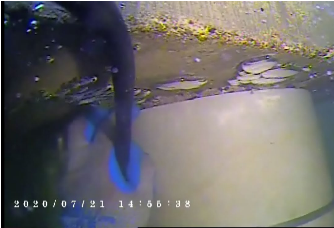
Image 7 – Interface of plastic UV protective wrap under concrete encapsulation (typical)
