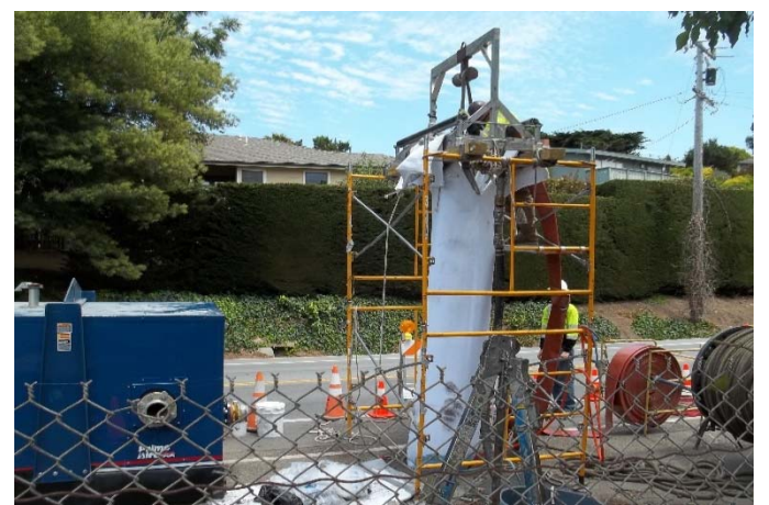
Photo: View CIPP Liner being installed
