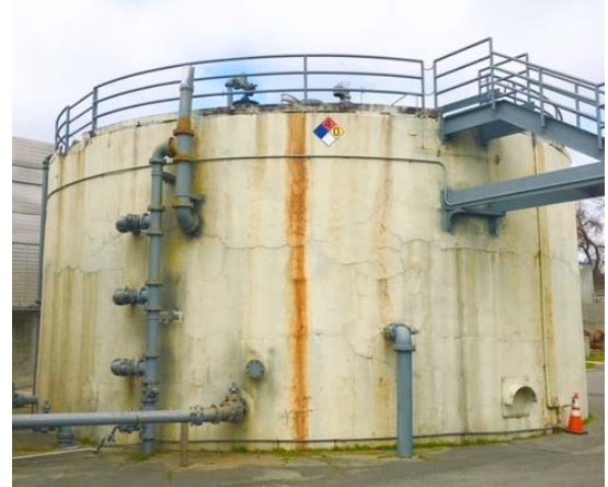
Photo: Old Digester No. 2
