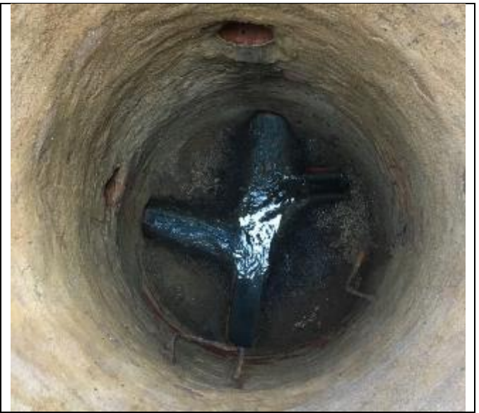
Photo: Inside of Sewer Manhole
