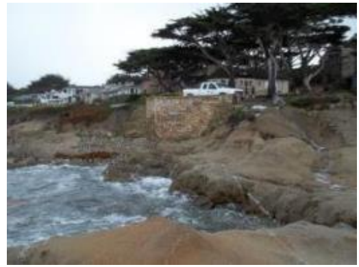
Photo: Looking at Pump Station Exterior
