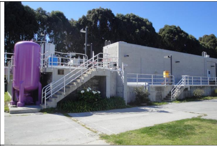
Photo: Exterior of Tertiary Building
