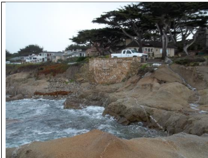
Photo: Looking at Pump Station Exterior
