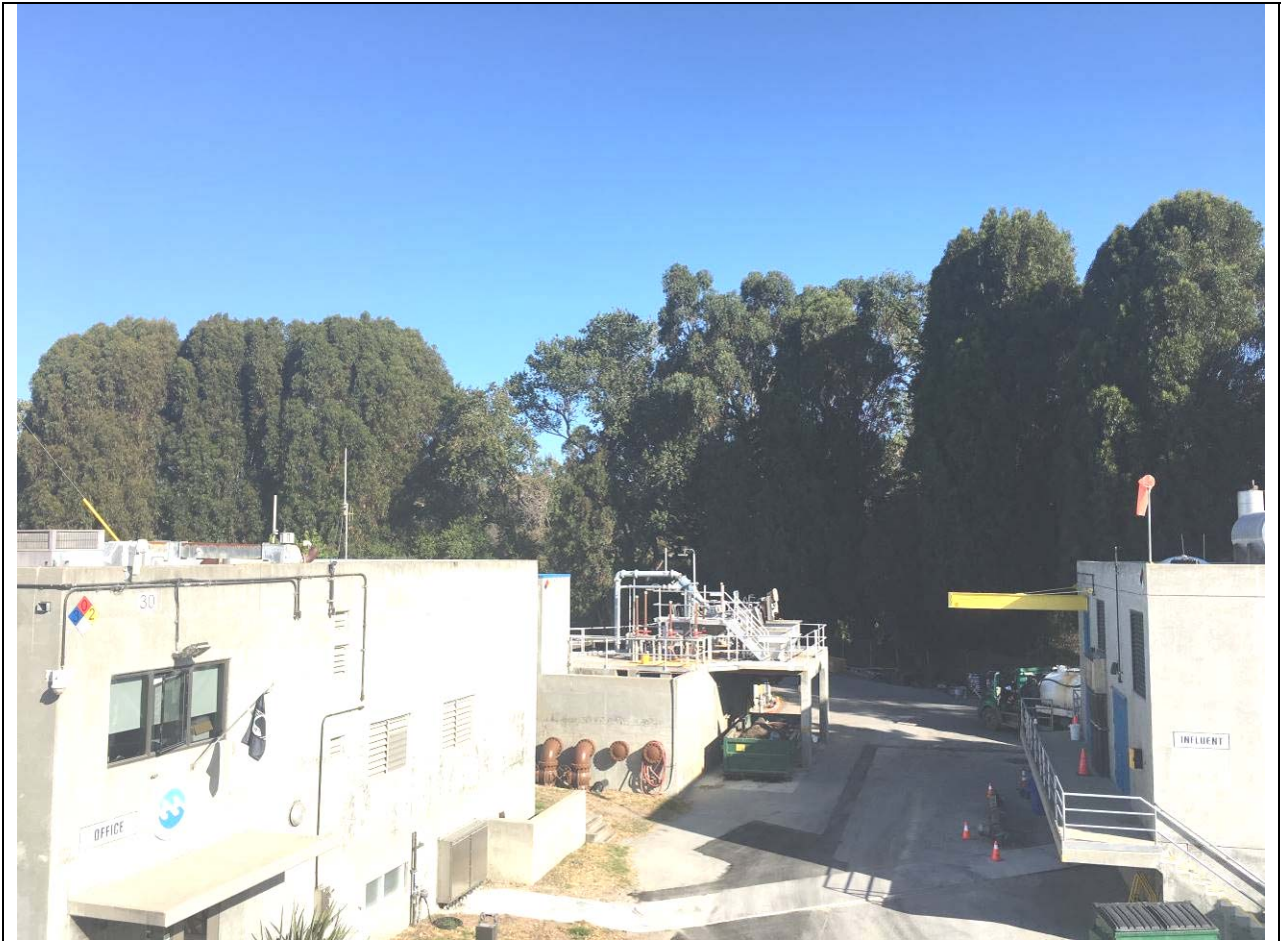
Photo 8: Taken from on top of an existing building inside the WWTP looking North at Northern property line. Note gap in eucalyptus filled in with cottonwood trees.
