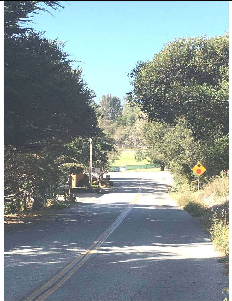
Photo 13: Taken from Atherton Dr Looking Southwest at the WWTP.
