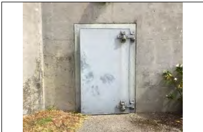
Photo: Old Flood Door in Headworks Basement
