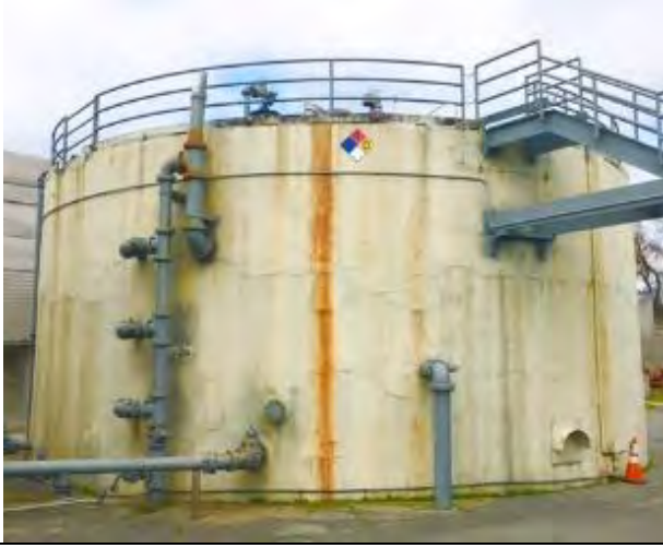
Photo: Old Digester No. 2
