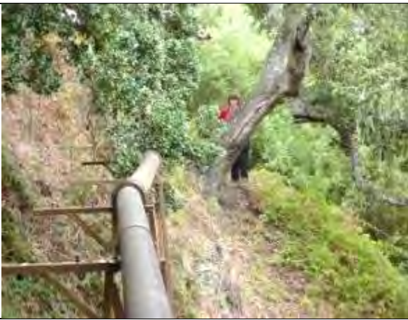
Photo: View gravity pipe in Carmel easement
