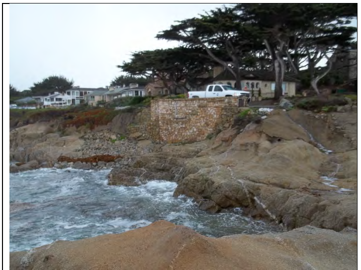
Photo: Looking at Pump Station Exterior
