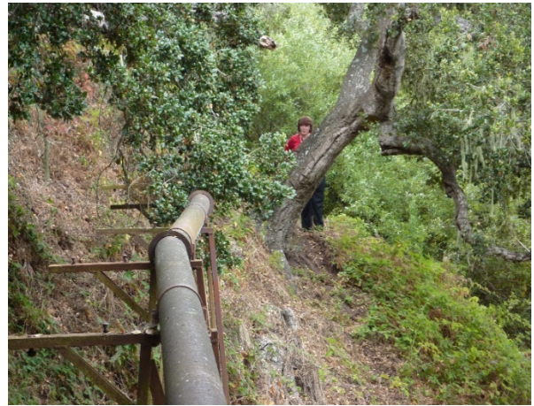
Photo: View gravity pipe in Carmel easement
