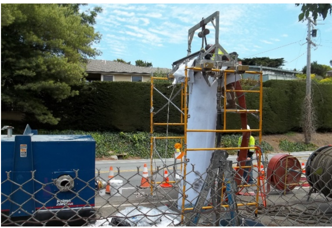
Photo: View CIPP Liner being installed
