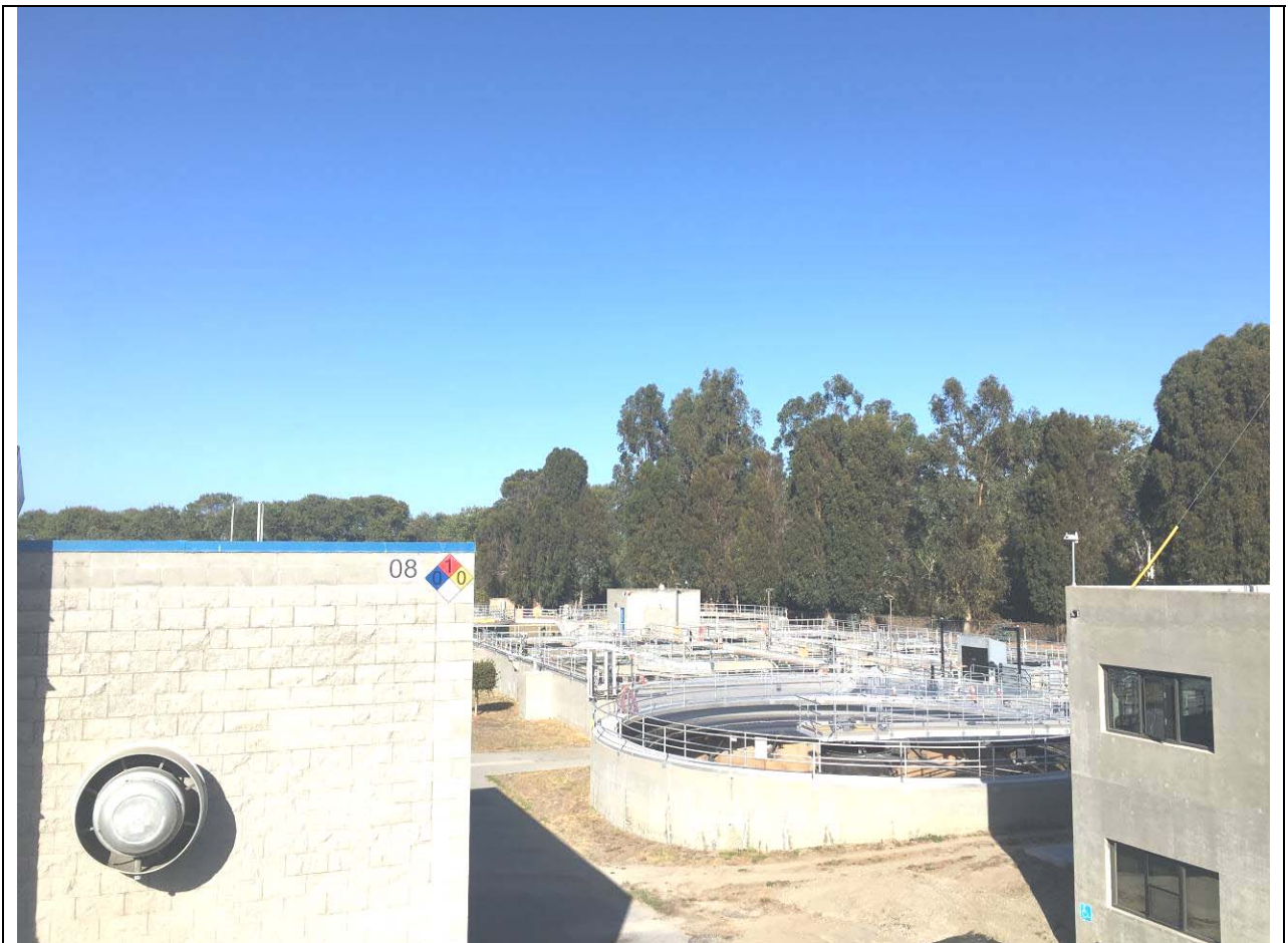
Photo 7: Taken from on top of an existing building inside the WWTP looking Northwesterly at Northern property line.
