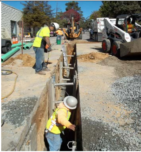
Photo: View of sewer line being replaced
