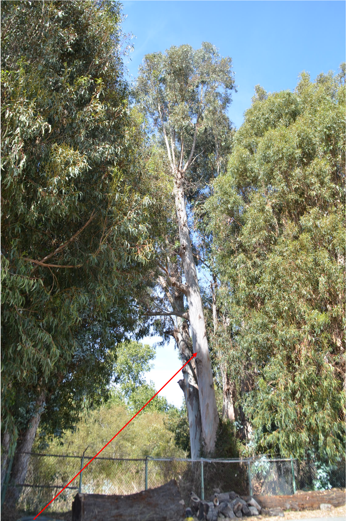
Large cluster of trees outside northwest corner. The upper portion has weakly attached branches prone to breakage
