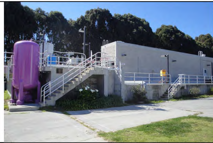
Photo: Exterior of Tertiary Building
