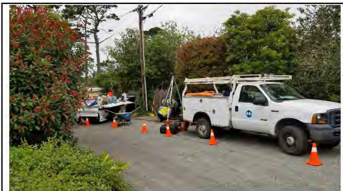
Photo: Pipe Repairs
