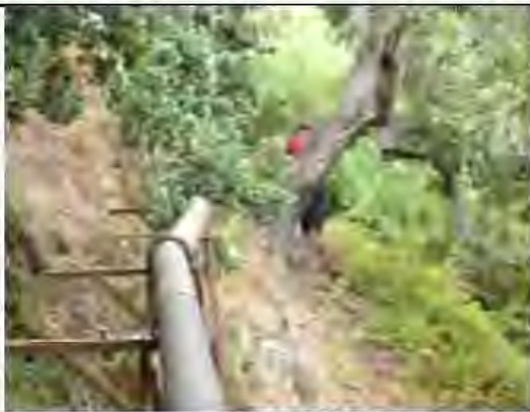
Photo: View gravity pipe in Carmel easement
