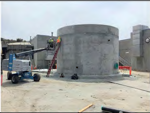
Photo: New Sludge Tank Under Construction
