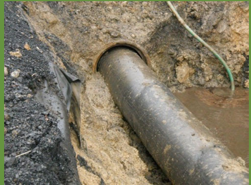
Photo: Slip-lining existing sewer main
