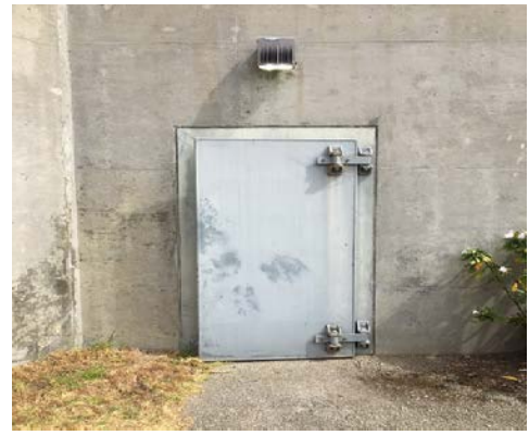
Photo: Old Flood Door in Headworks Basement
