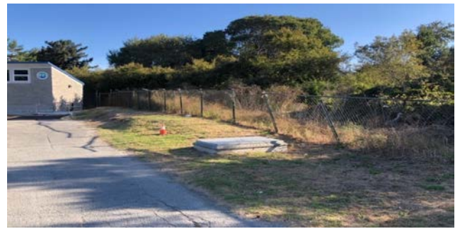
Photo: Eastern side of Perimeter Fence
