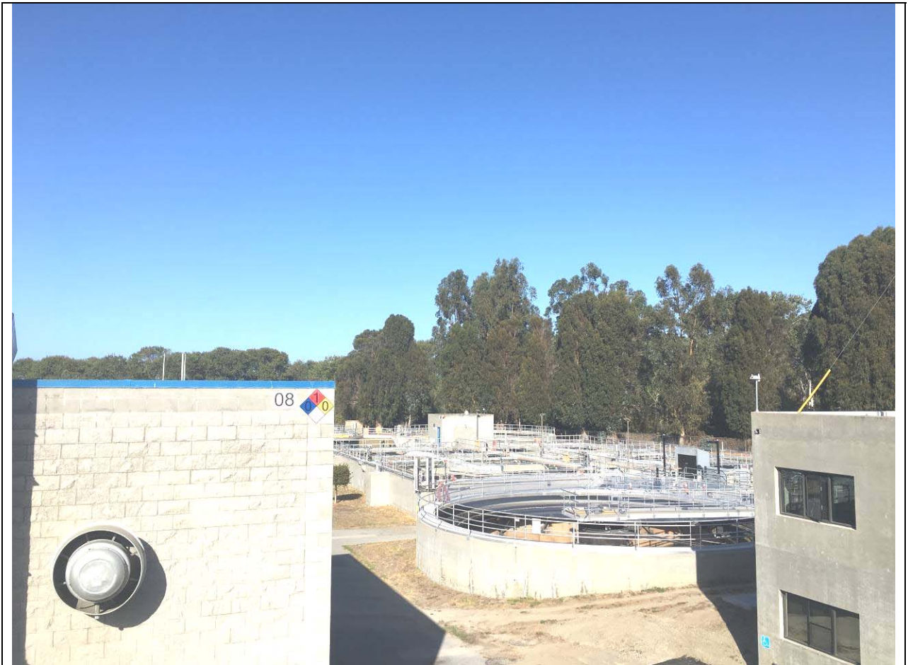
Photo 7: Taken from on top of an existing building inside the WWTP looking Northwesterly at Northern property line.
