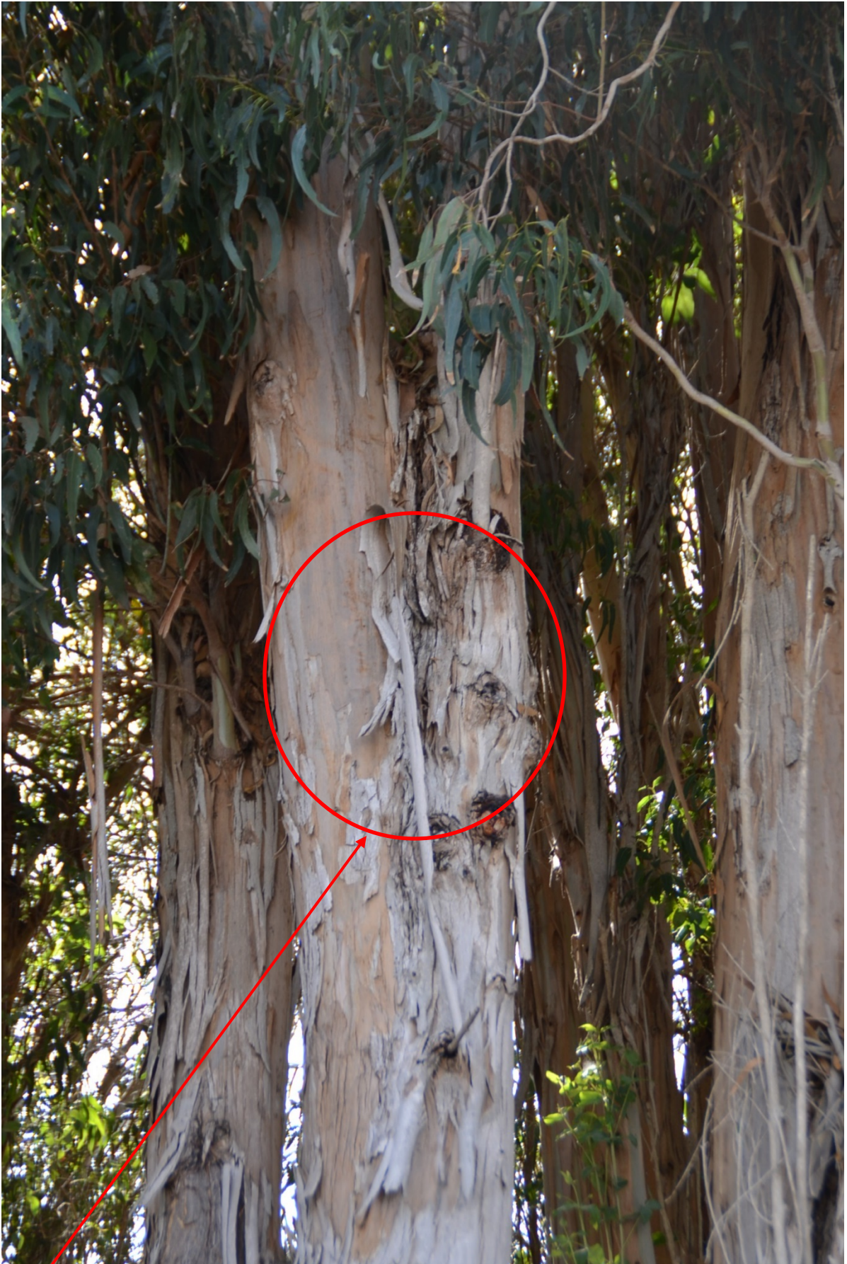
A number of trees have included bark at unions; this one appears to be separating and need attention
