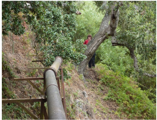
Photo: View gravity pipe in Carmel easement
