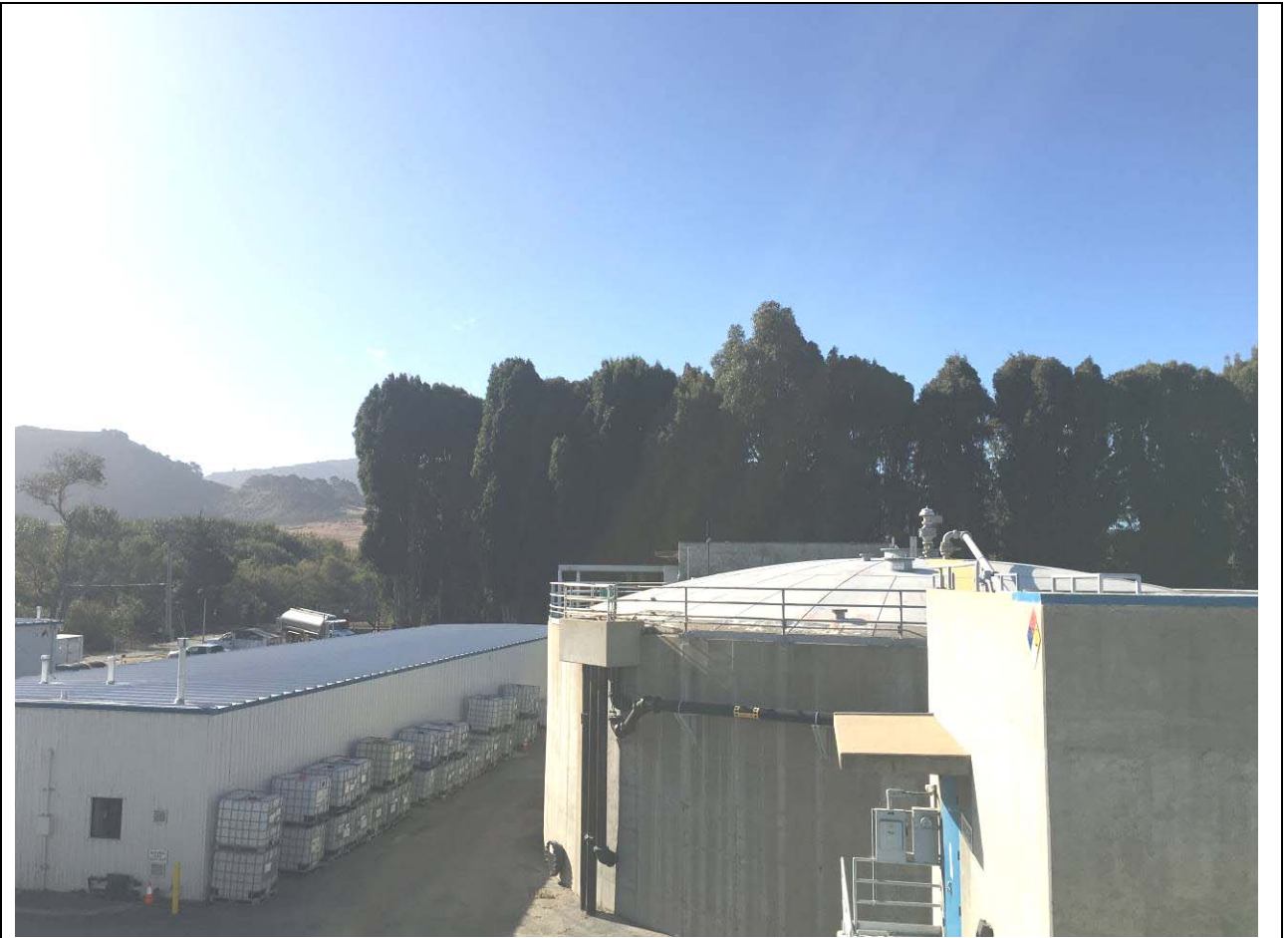
Photo 1: Taken from on top of an existing building inside the WWTP looking Southeasterly at southern property line.
