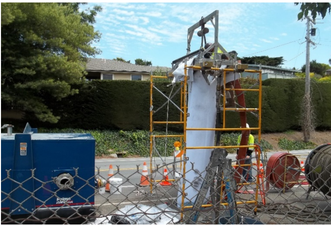
Photo: View CIPP Liner being installed
