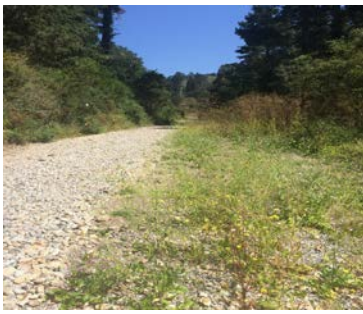
Photo: View of portion of Hatton Canyon Access Road that was repaired to allow access for construction equipment
