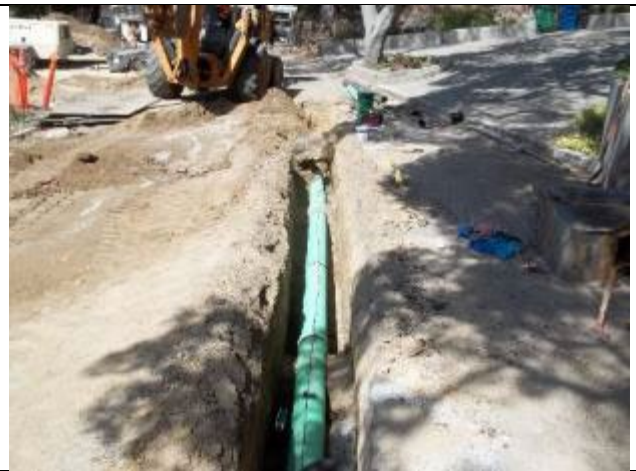
Photo: Sewer Line Repair
