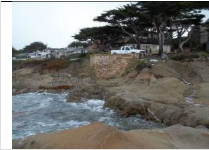
Photo: Looking at Pump Station Exterior
