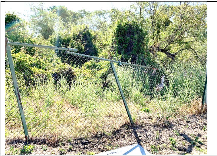
Photo: Existing Dilapidated Fence
