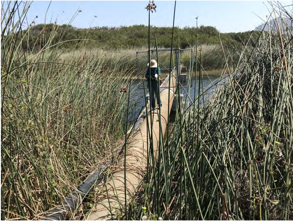
Figure 5: View of Existing Pipelines crossing Carmel River Lagoon
