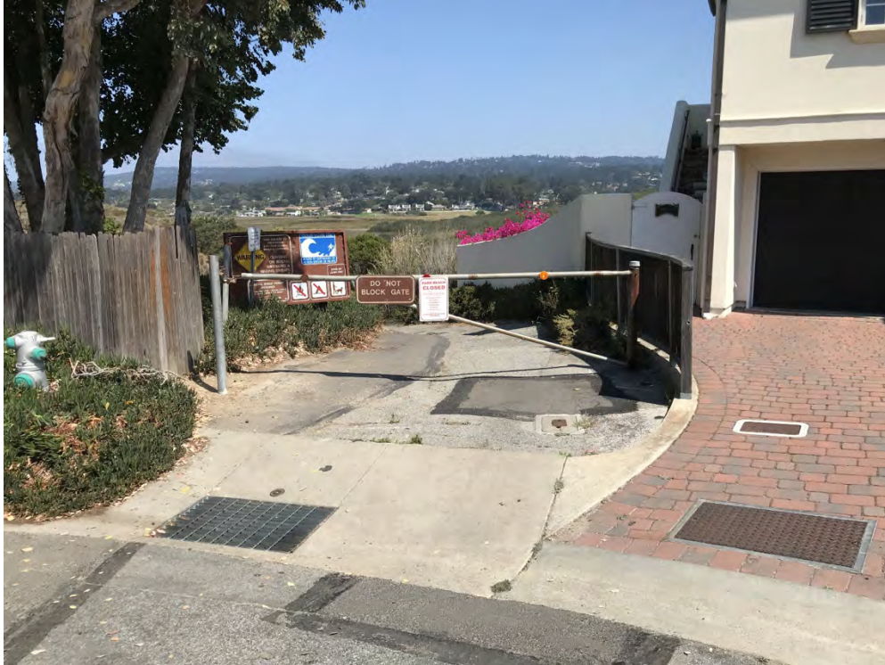
Figure 7: View of CAWD Pump Station Access Road from Calle La Cruz
