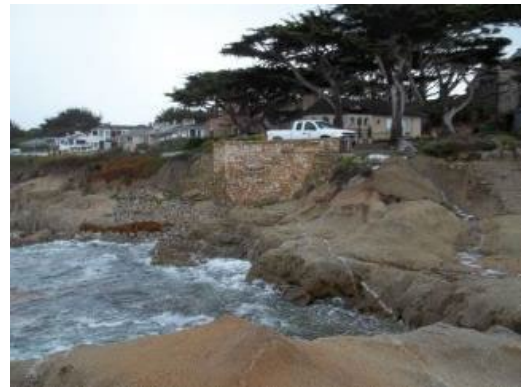
Photo: Looking at Pump Station Exterior
