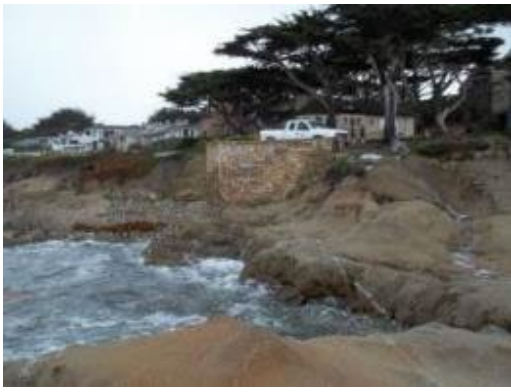
Photo: Looking at Pump Station Exterior
