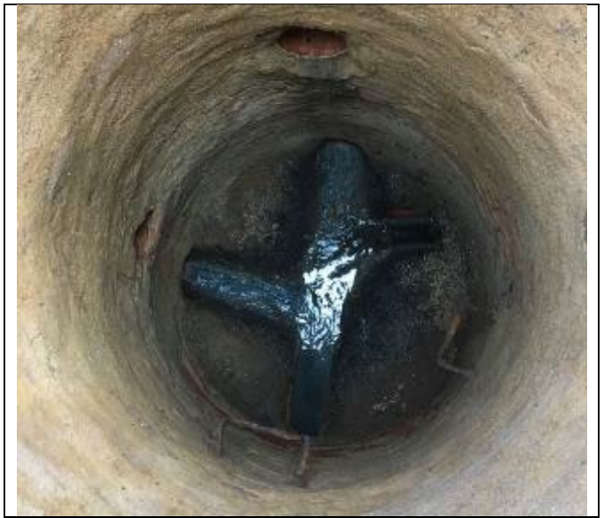
Photo: Inside of Sewer Manhole
