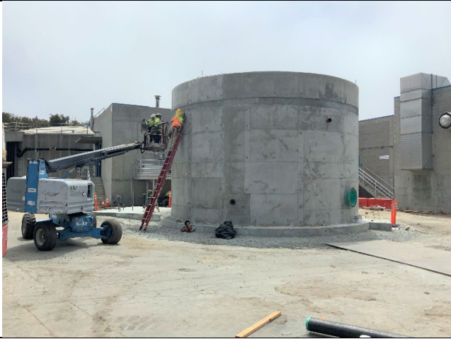
Photo: New Sludge Tank Under Construction
