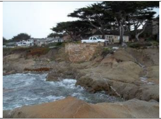
Photo: Looking at Pump Station Exterior
