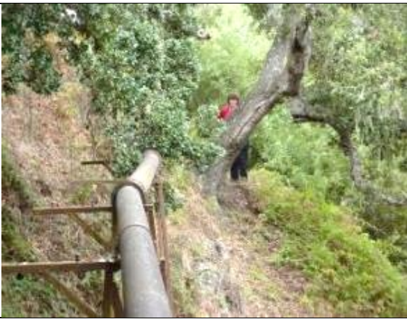
Photo: View gravity pipe in Carmel easement
