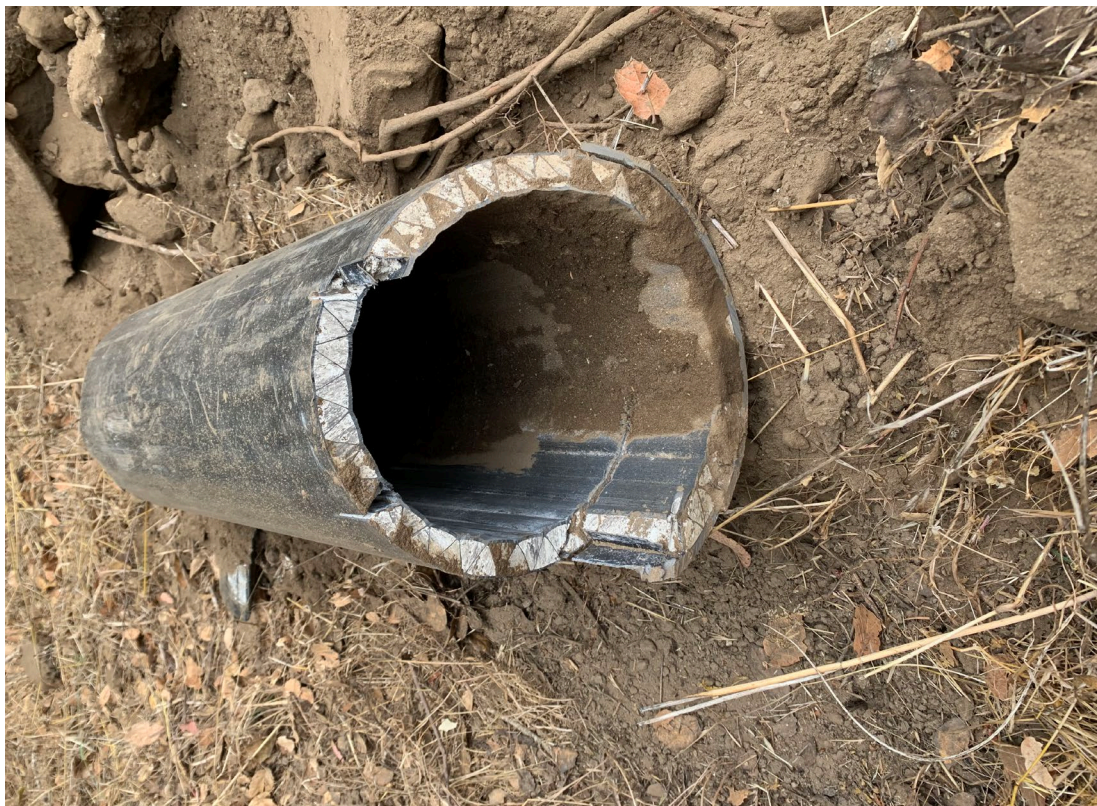
Photo No. 1 -View of Truss Pipe
