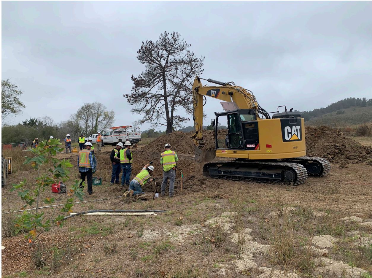
Photo No. 3- View of Trenching in Palo Corona Park
