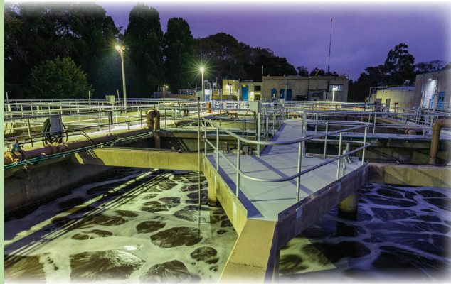
NIGHTWATCH AT THE PLANT In adherence with COVID-19 guidelines, CAWD staff are split into day and night shifts to ensure that we have skilled plant operators even if one shift has to quarantine.
