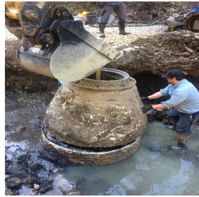
Photo: View of a temporary repair of a manhole in Hatton Canyon
