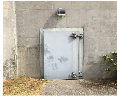
Photo: Old Flood Door in Headworks Basement
