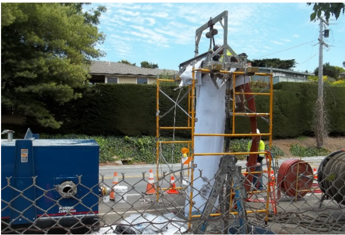
Photo: View CIPP Liner being installed
