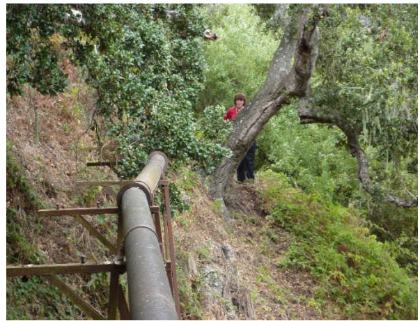
Photo: View gravity pipe in Carmel easement
