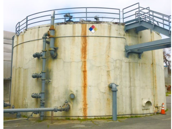
Photo: Old Digester No. 2
