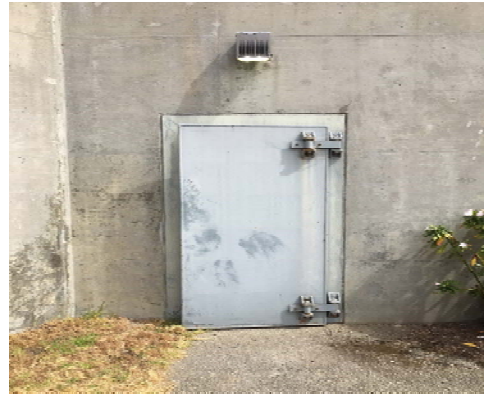
Photo: Old Flood Door in Headworks Basement
