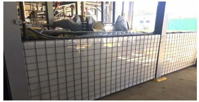
Photo: Sound Barriers partially installed around High Pressure RO Pumps
