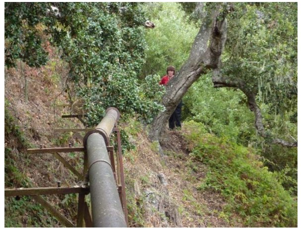
Photo: View gravity pipe in Carmel easement
