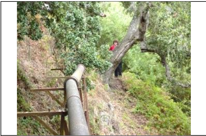
Photo: View gravity pipe in Carmel easement
