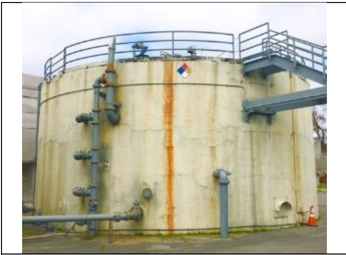
Photo: Old Digester No. 2
