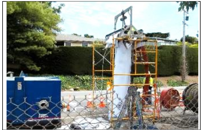
Photo: View CIPP Liner being installed
