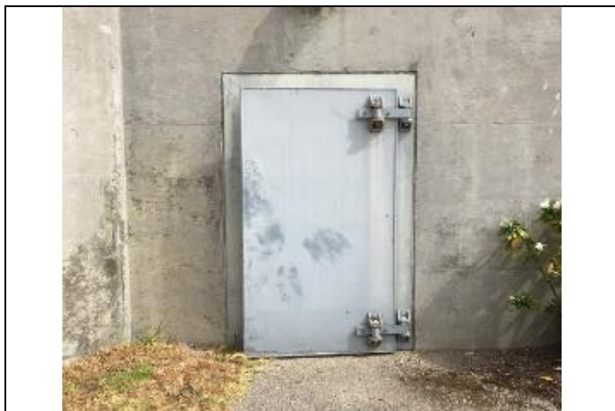
Photo: Old Flood Door in Headworks Basement
