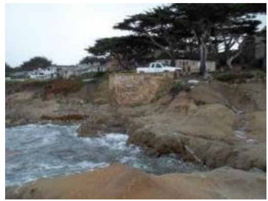
Photo: Pump Station Exterior
